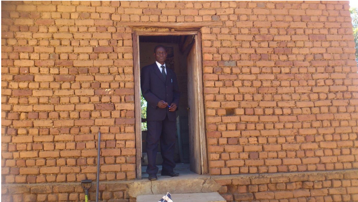
Plate 24: State of Headmaster's Office
