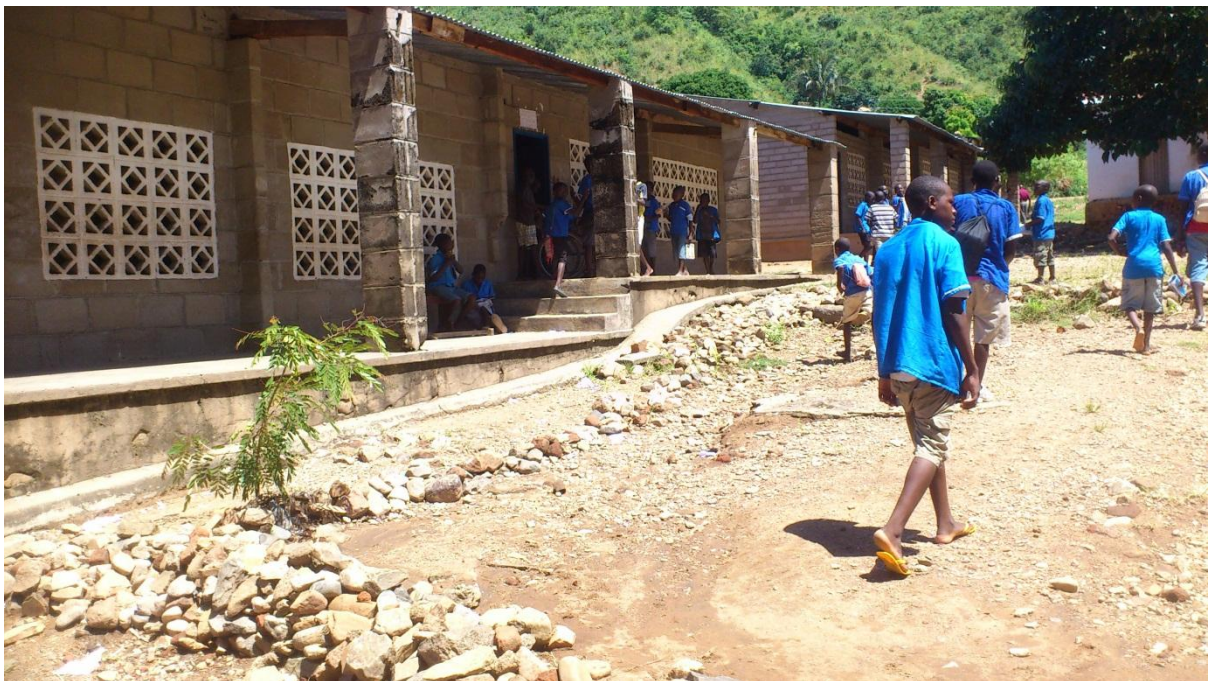
Plates 22: Poor State of Outside School Grounds
